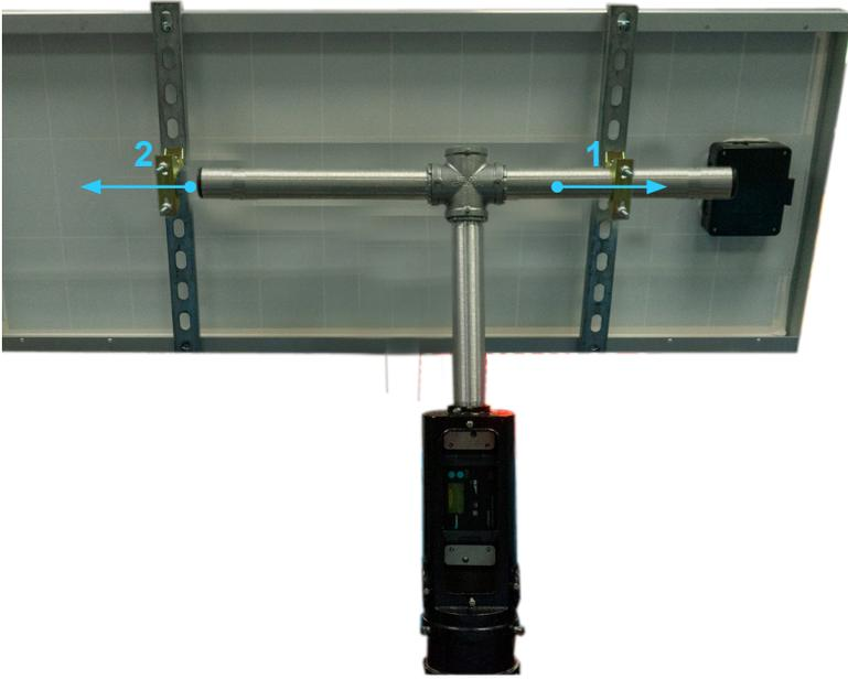
2. Slide the panel the opposite direction to capture both serrated clamps on the mounting structure's horizontal pipes
